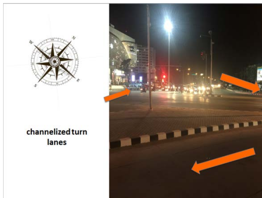
Figure 27 Image of channelized turn lanes at the intersection. A compass to the left of the photo provides the orientation and arrows point to indicate traffic flow.
