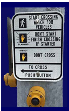
Figure 19 Picture shows a pole with pushbuttons mounted on it under a sign explaining how to use the sign (white silhouette of walking person means “Start crossing, watch for vehicles”; flashing orange hand means “don’t start, finish crossing if started”; steady orange hand means “don’t cross.” An arrow pointing to the left says “to cross, push button.”
