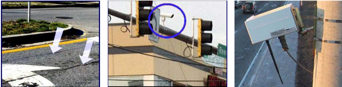
Figure 16 A series of three images (left to right) induction loop shows lines in the pavement of the street, camera mounted on signal, and radar mounted on a street pole.
