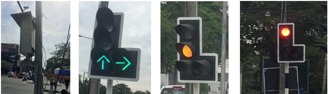
Figure 35 A series of four photos (from left to right): a controller box, signal head showing proceed straight ahead and right turn. a signal head showing
